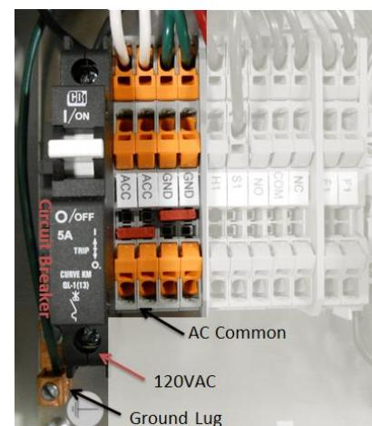
**Power Wiring.** The M.E.I. High Level Float Alarm should be provided with a clean 120VAC, 60Hz, single phase circuit. The incoming power must be provided with a circuit breaker or a disconnect switch with fuses in accordance with NEC and all local codes. Minimum wire size is 14awg.
